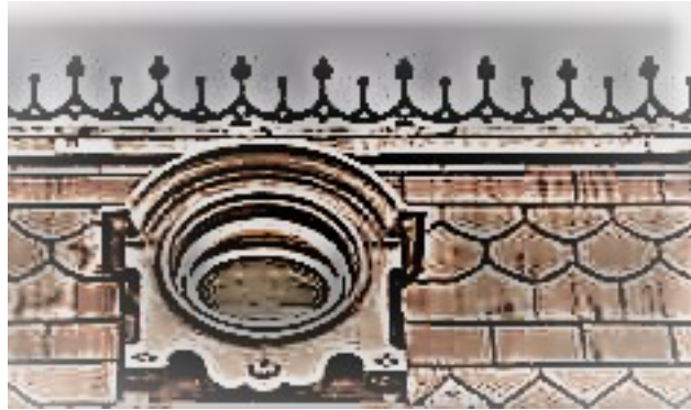
Example of an ornamental iron roof balustrade.
