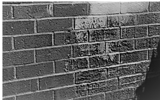
Effects of sandblasting on brick surfaces.
