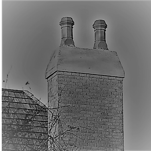
Example of clay chimney caps.
